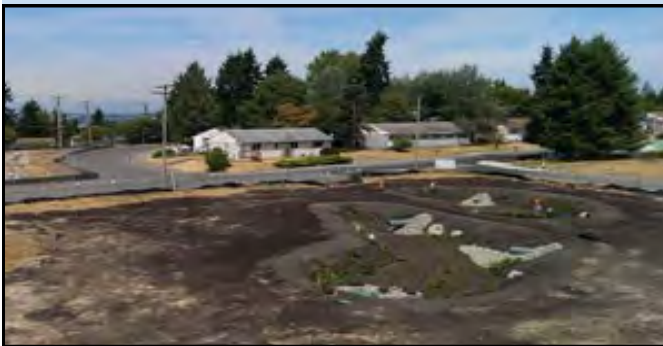
Sunset Terrace Regional Stormwater Facility
