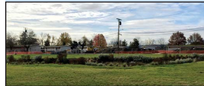
Sunset Terrace Regional Stormwater Facility
